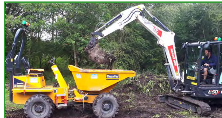
Excavating new pond at Hollymoor Grove, HCP
